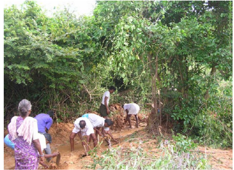
Maintaining existing structures
