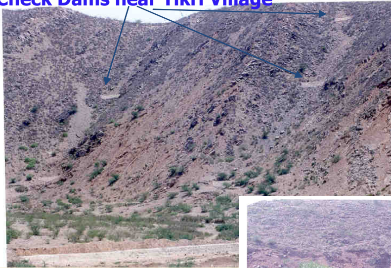
Check Dams near Tikri Village
