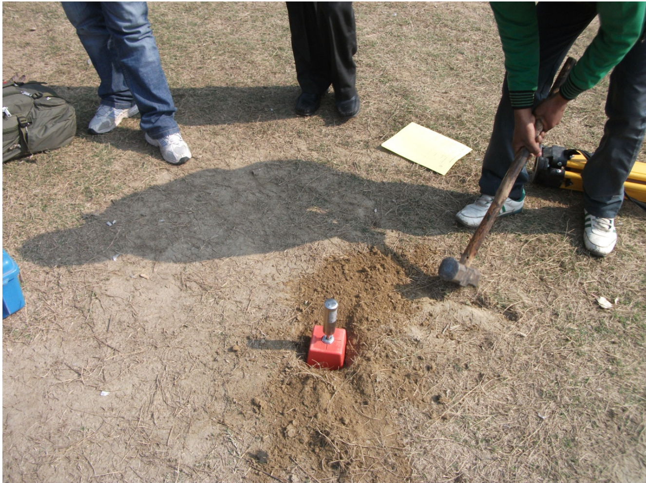
Installing Secondary point
