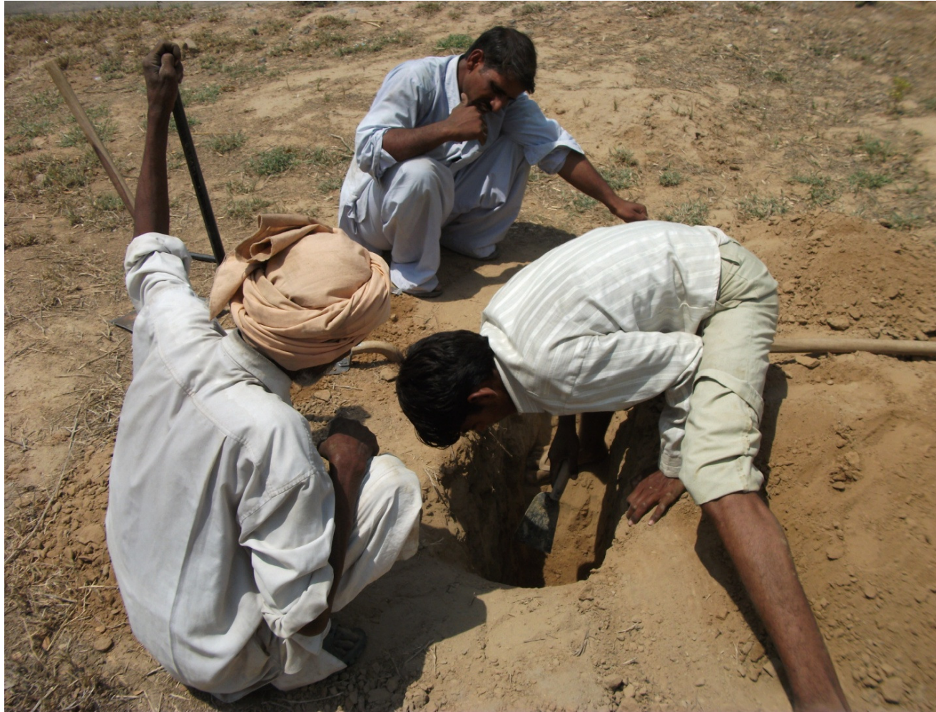
Digging the pit for central pillar of primary point
